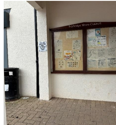
3. No smoking signage externally
