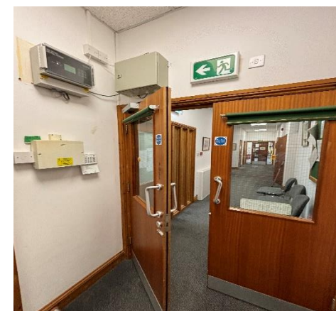
32. Check fire alarm provision
