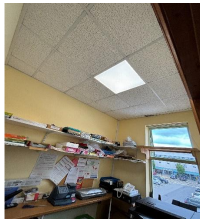
31. Check fire alarm provision
