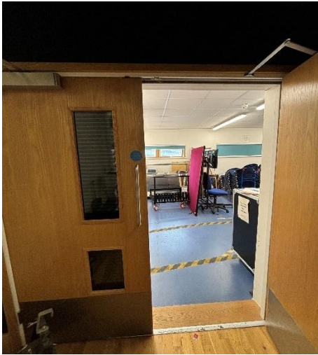
41. Stowford Hall exit to control room
